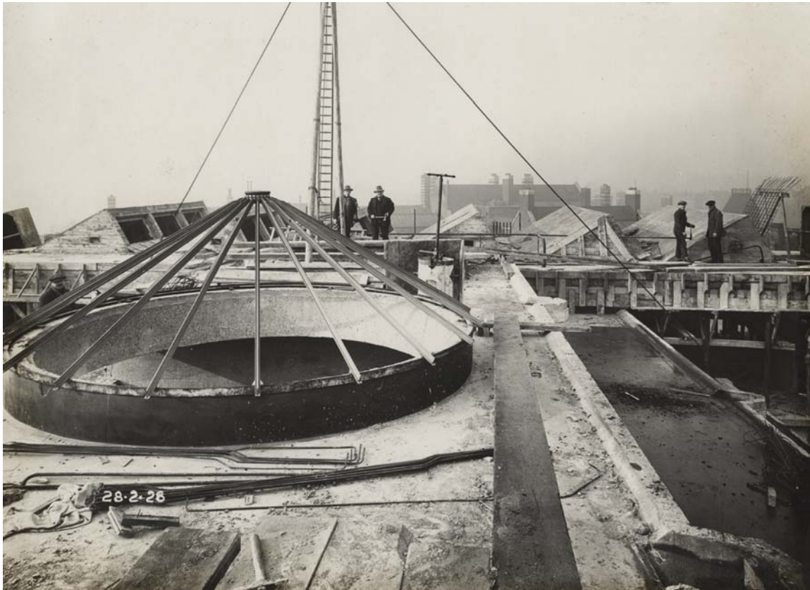
4.19 Above Skylights on top of the roof slabs of the Royal Horticultural Hall under construction. From RHS, Lindley Library.
