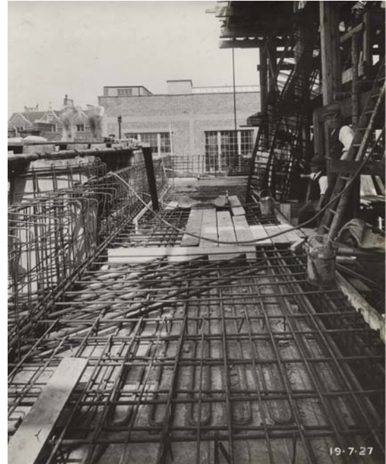
4.16 The North Aisle's Roof Slab under construction, photographed in July 1927. The aisles' slabs act as 'transfer beams' carrying the thrust of the arches before transferring it to the ties of the end walls. From RHS, Lindley Library.
