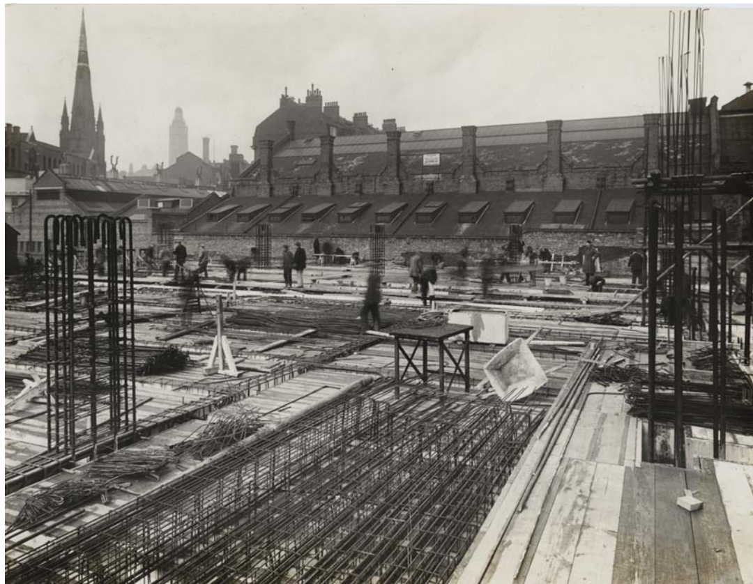
4.17 Rebars of the Royal Horticultural Hall's Ground Floor in construction. The photograph was taken from the rear towards the front of the building. From RHS, Lindley Library.
