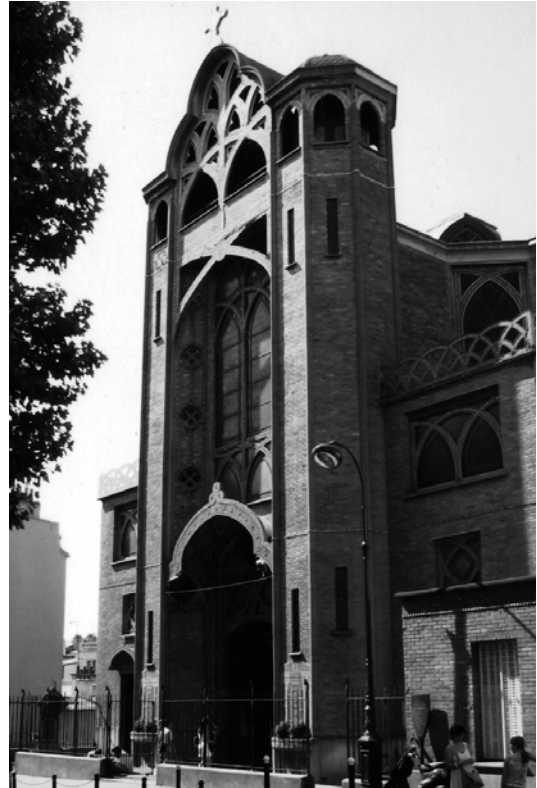
1.6 The first reinforced-concrete church of St. Jean de Montmartre, Paris, France, built in 1894 and completed in 1904, photographed in 2008. Anatole de Baudot, architect. Paul Cottancin, engineer. 1894-1904.
