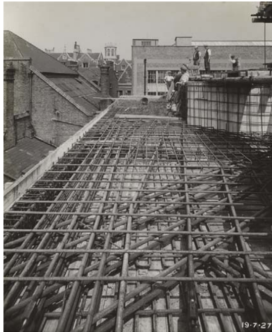
4.13 Left Rebars of RHH's main arch and the north aisle's roof slab in construction, photographed in July 1927. The extra reinforcing bars, laid diagonally, were cast into the aisles' roof slabs to carry the thrust of the main arches and led to the change of the skylight's shape. From RHS, Lindley Library.
