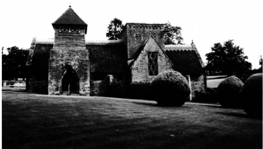
3.14 All Saints' Church, Brockhampton, designed by W.R. Lethaby in 1901-02. The composite nature of roof construction mixes thatch with concrete, most unusual for a new church built in the early 1900.
