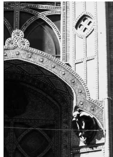
1.13 Ceramics Tiles above the Doorway of St. Jean de Montmartre, photographed in 2008. De Baudot's use of non-structural materials to conceal the concrete construction did not follow the law of structural rationalism. Yet does this invalidate the church as a 'building'?
